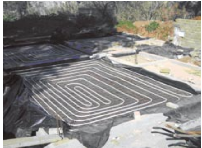
Plancher chauffant
